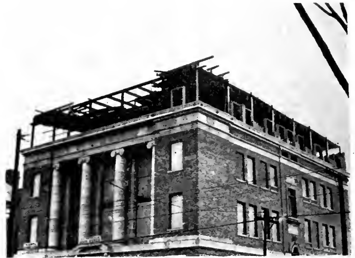
Fig. 4.—Administration Building, Toronto. Erection Progress Jan. 6.
